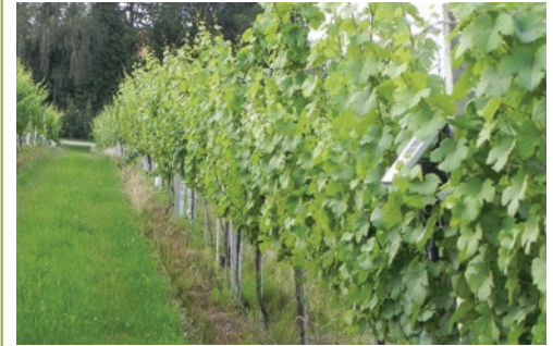
Node installation with solar panels in Slovenia
